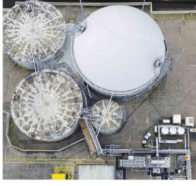
city to the neighbouring wastewater treatment works or the public grid. The heat is used to heat the digesters and pasteurise the digestate on site. In addition, the process produces 1,886 tons of solid digestate for compost production (20-25% dry matter) and 37,611 tons of liquid digestate for crop production (3-4% of dry matter) a year. These are impressive figures, showing what state-of-the-art waste processing technology is capable of.
