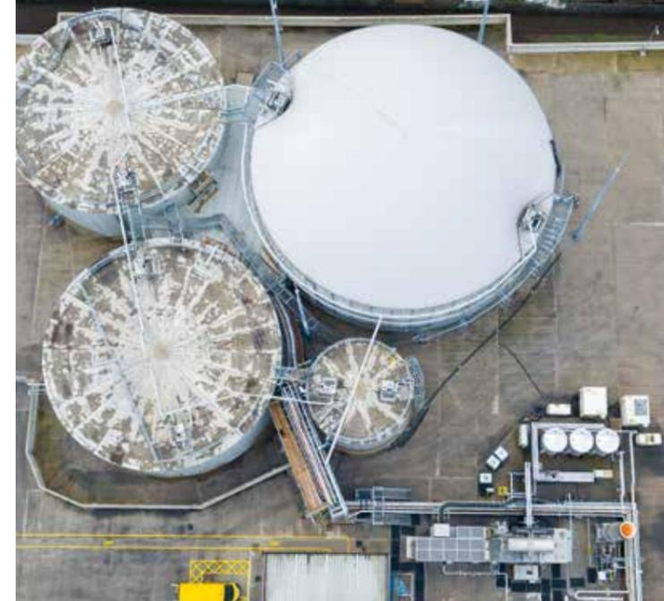
city to the neighbouring wastewater treatment works or the public grid. The heat is used to heat the digesters and pasteurise the digestate on site. In addition, the process produces 1,886 tons of solid digestate for compost production (20-25% dry matter) and 37,611 tons of liquid digestate for crop production (3-4% of dry matter) a year. These are impressive figures, showing what state-of-the-art waste processing technology is capable of.
